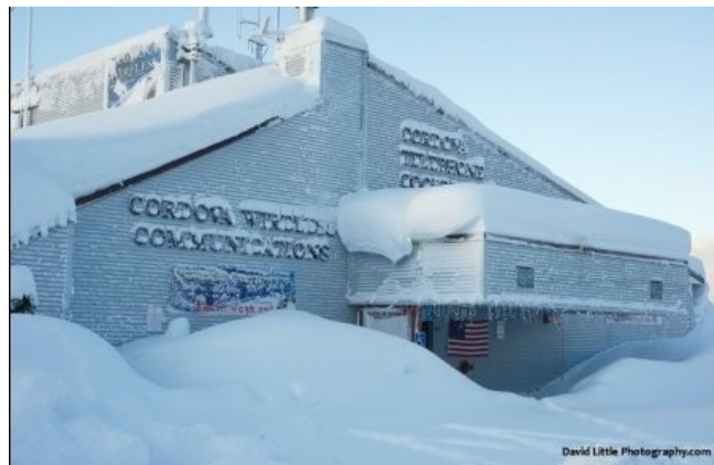
Telephone company office
